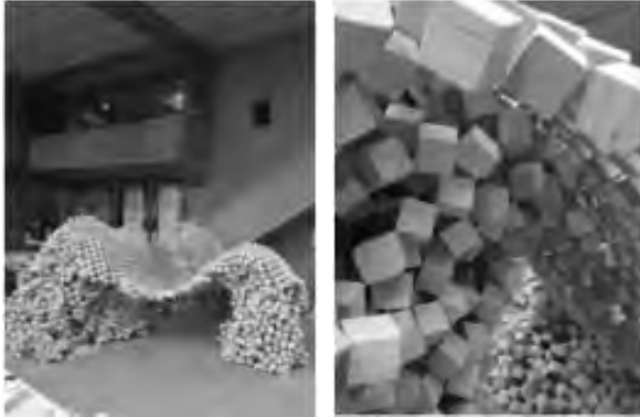
Fig 12. ? cube. 60 mm cubes made of hemlock spruce connected by “?” shaped eye bolts. The structure gradually changes from a hard structure at the base to a membrane-like structure on the roof. The distance between nodes is the dimension of the cube elements of dimension x , x , x\sqrt{2} , x\sqrt{3} . Design & Construction : Ken Yokogawa Laboratory, Nihon University. Structure: Jun Sato.
