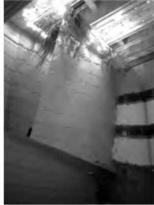
Fig 10. Balloon. Aluminium "balloon" of height 14m, weighing roughly 1 tonne. The balloon has an aluminium lattice frame skeleton and is filled with helium gas. Architect : Junya Ishigami. Structure : Jun Sato.
