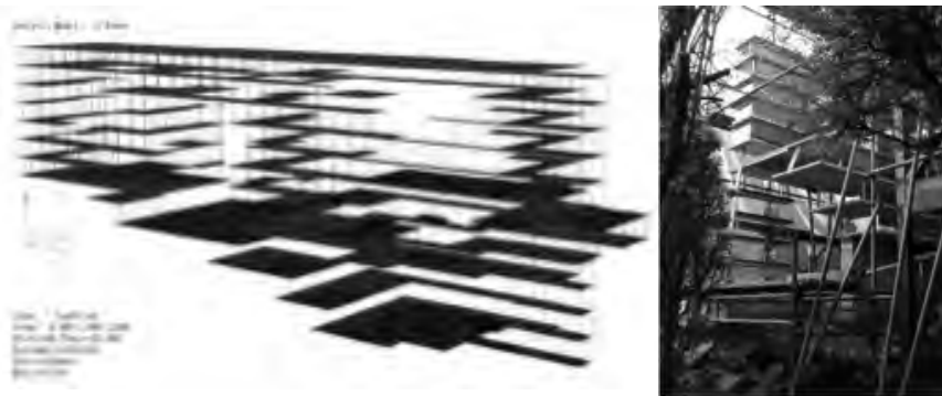
Fig 2. Iz House, Stacked structure of glass and acrylic resin walls. Architect: Sou Fujimoto, Structure : Jun Sato.
