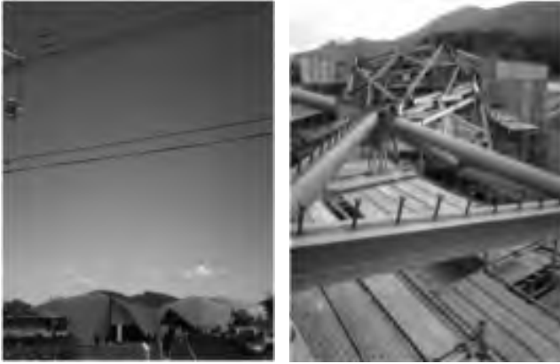
Fig 14. Community Centre, Kawatana Onsen. Polyhedral form generated by moving nodes. Development of software for form finding under several load combinations such as gravity, seismic load, snow and wind. The parameter to be focused will be safety ratio, energy absorption. Architect: Kengo Kuma, Structure: Jun Sato.
