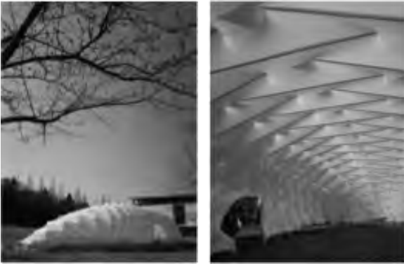
Fig 11. MOOM (Membrane Oom). Tensegrity structure composed of membrane and aluminium pipes. Length 26 m, Span 8 m. Design & Construction : Kazuhiro Kojima Laboratory, Tokyo University of Science. Structure : Jun Sato.
