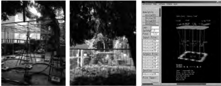
Fig 1. Proposal for Transparent Glass, Resin Structure, EXTREME NATURE , Venezia Biennale 2008. Slender, rigid frame structure using high strength steel with glass walls acting as tension elements. The heat camber method used is important in forming the camber which reduces deflections as well as bending stresses. Development of Manual Form Finding Software to find optimized location of columns. Architect : Junya Ishigami, Structure : Jun Sato
