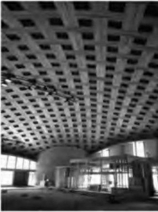
Fig 8. Ashikia Community Hall. Thin laminated timber structure inspired by the structure of a bamboo basket. Architect : Akiko Takahashi, Hiroshi Takahashi / Workstation, Structure : Jun Sato.
