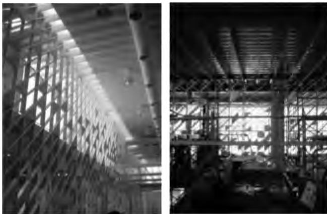
Fig 4. Research Building, Hakodate Future University. Steel mesh structure composed of vertical and diagonal elements Architect : Riken Yamamoto. Structure : Jun Sato.
