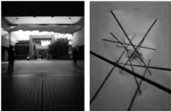
Fig 13. “Big Art” in the Archi-neering Exhibition. Tensegrity structure composed of a membrane supported by carbon (CFRP) pipes. Designed and Constructed by about 15 students. Structure : Jun Sato et al.
