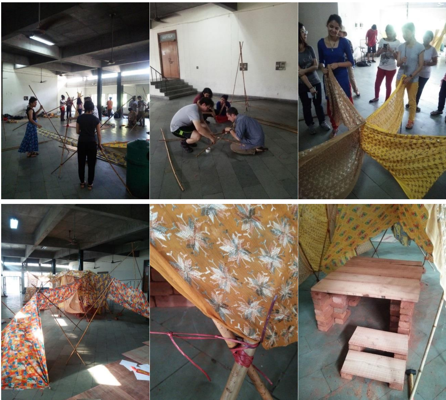
Day 2nd: Studies on bamboo frames, branching membrane structure, brick and board for lifted platform.
